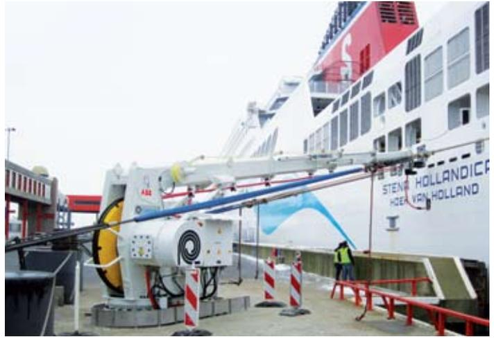
Connecting Stena Hollandica to the local grid
