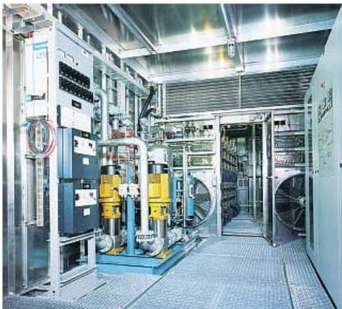
Fig 8. Example of a static converter; source ABB
